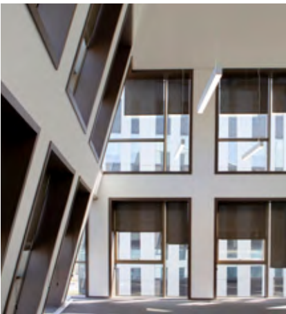
PREMIUM PLUS ROLLER SHADES WITH REFLECTIVE FABRIC AND 15° INCLINED INSTALLATION.
