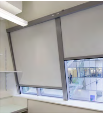
INCLINED B-BOX ROLLER SHADES WITH SIDE CHANNELS AND BLACKOUT FABRIC (MAXIMUM OPACITY).
